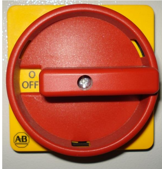
Figure 6. Main isolator switch in the "OFF" position
